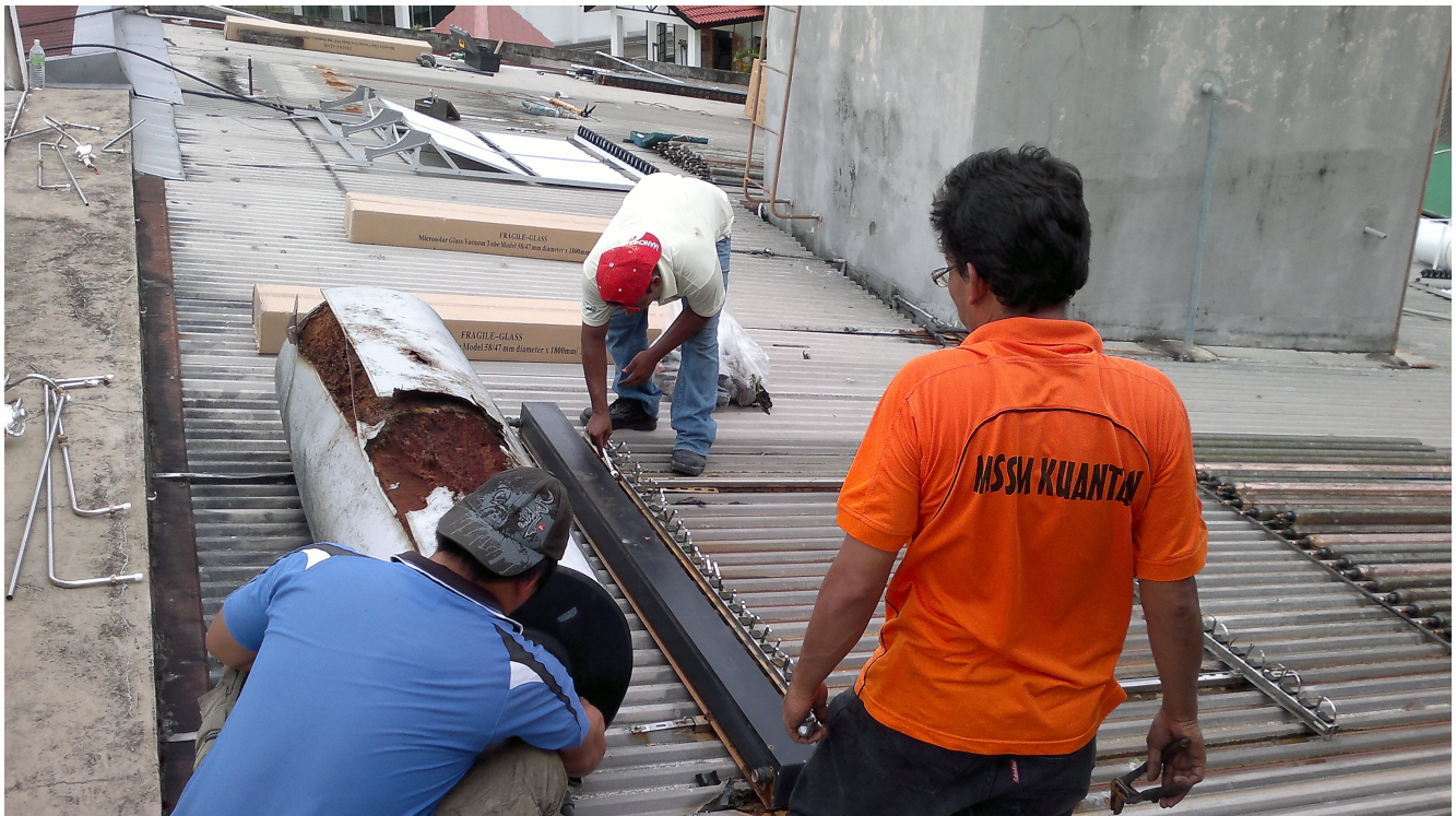
Removing clogged up 7 years old heat pipe solar heaters.
