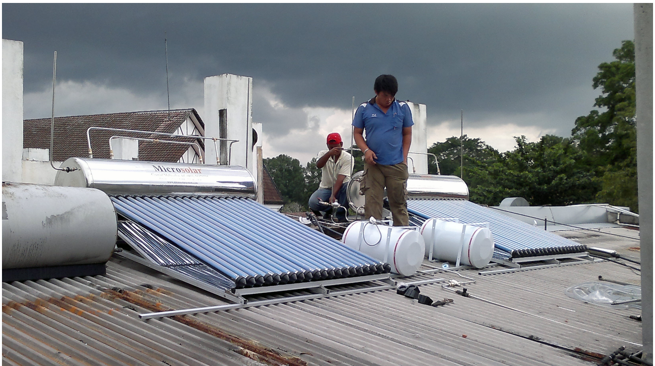
Installing new Microsolar Coaxial Multivalve M70VTHE.
